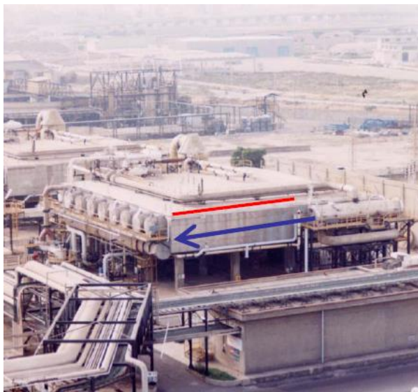
Figura 22 - Gela, 4x14400m 3 /dia (Fonte: Promotion of Renewable Energy for Water production through Desalination)
