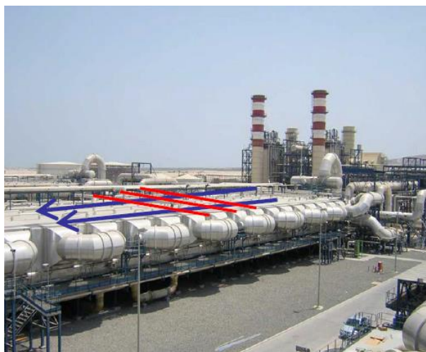
Figura 21 - Shuweihat, 76500m 3 /dia (Fonte: Promotion of Renewable Energy for Water production through Desalination)
